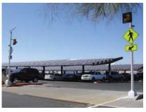
pany recently added several kilowatts of solar roofing to its covered parking area at its main facility in Phoenix. The grid intertie system produces electricity from the sun during the day and pushes it back onto the grid to offset the company's energy use.
